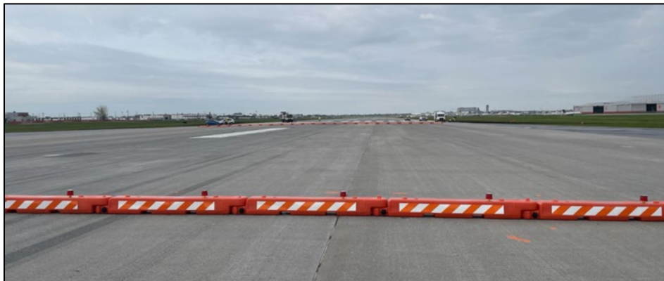
Figure 3. Low profile barricades with obstruction lights
