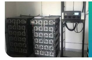
8-hour/48-hour Emergency Back-up Battery System
