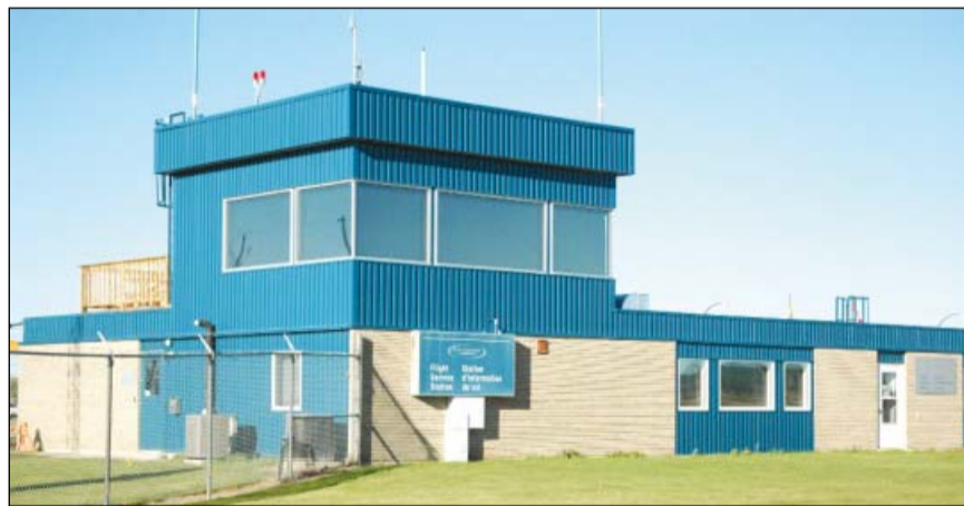
The Nav Canada flight service station at the Prince Albert airport.
