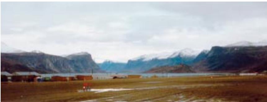
Photo 3-1 - Looking northeast from Pangnirtung runway
