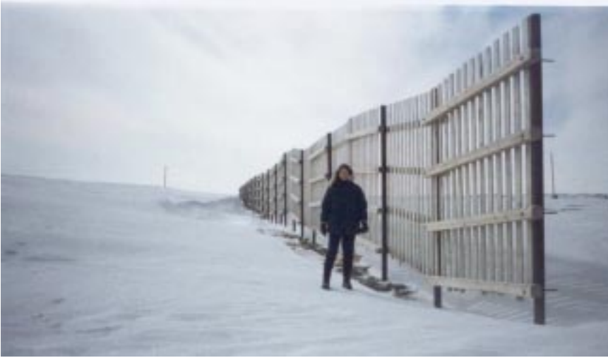
Photo 3-7 - Snow fence at Rankin Inlet
