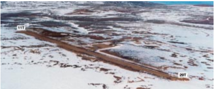
Photo 5-7 - Nanisivik runway, looking north
