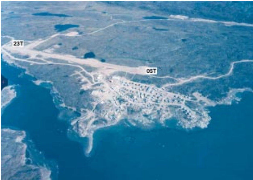
Photo 5-20 - Kugaaruk community and airstrip, looking southeast
