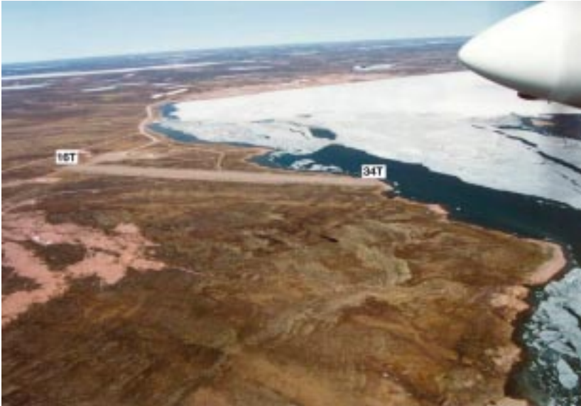
Photo 5-1 - Baker Lake, runway (foreground) and community (background), looking northwest
