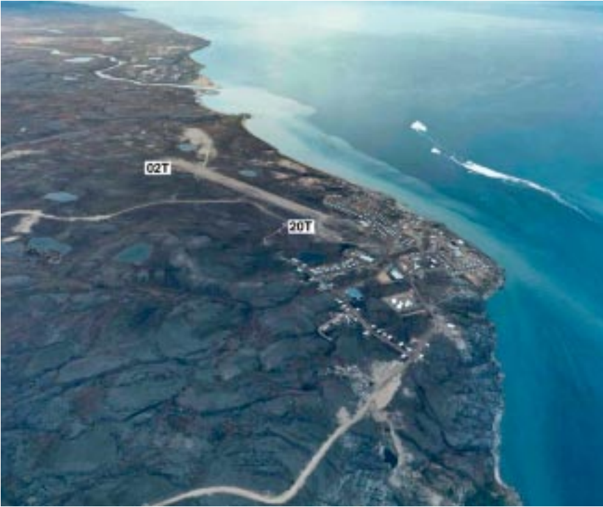
Photo 5-8 - Pond Inlet, looking west
